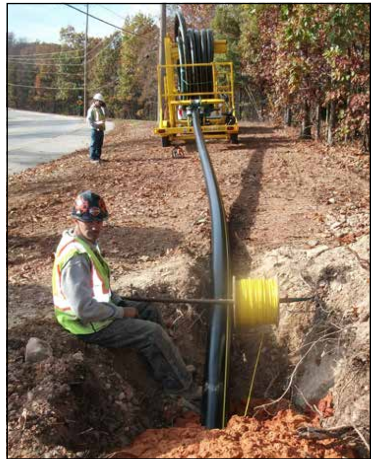
Summit Natural Gas is in the process of installing service lines in several areas around the Lake of the Ozarks area, including Horseshoe Bend. Nancy Zoellner-Hogland photo.
