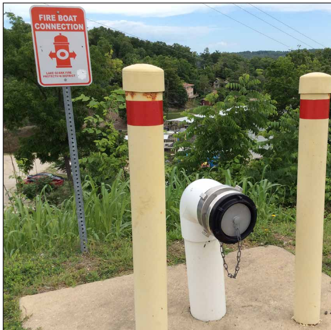
Dry hydrants don't look much like the traditional fire plugs but they serve the same purpose. Nancy Zoellner-Hogland photo.
