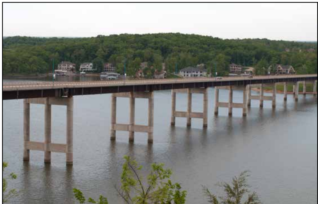
When the Lake of the Ozarks Community Bridge was completed and opened to traffic on May 1, 1998, the peninsula on the west end of the bridge extended to the second set of piers. Intense wave action has been blamed for washing away more than 50 feet of that land. File photo.
