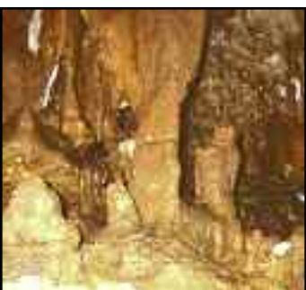
The horizontal crack in this column is evidence of an unknown shift—possibly an earthquake. Photo by Michael Gillespie.
