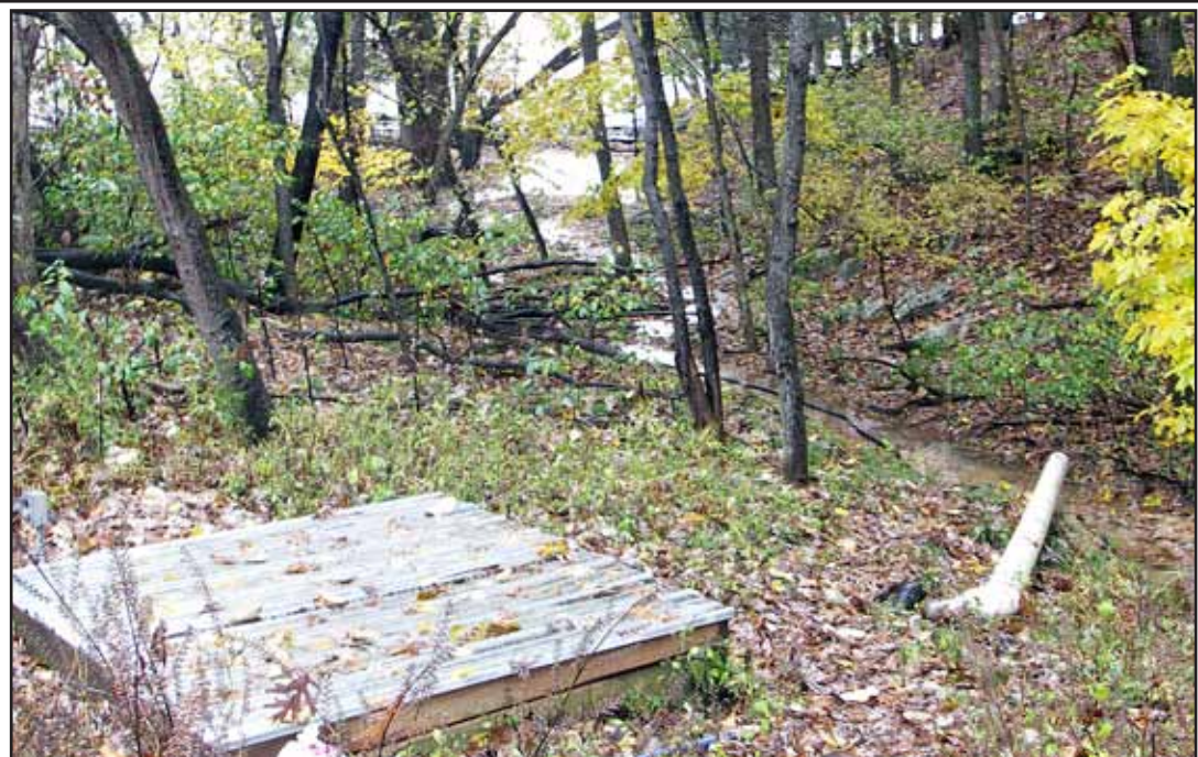
This unmarked white PVC pipe discharges the water into a small ditch that drains into Lake of the Ozarks. According to the permit issued for this seemingly forgotten treatment facility, all outfalls must be clearly marked. Nancy Hogland photos.
