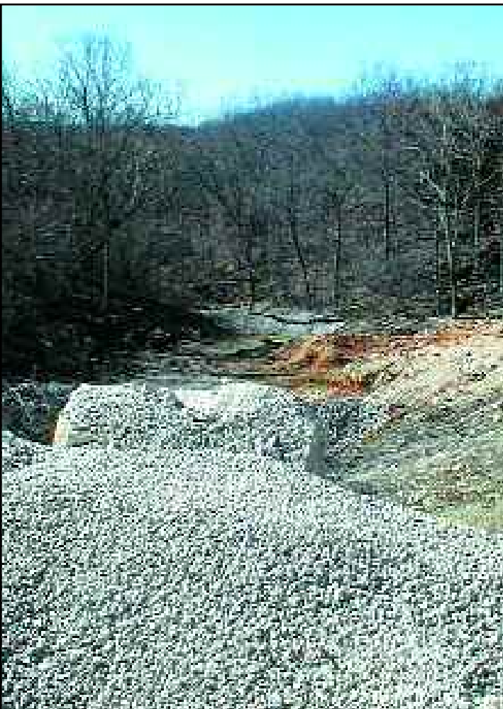
Four aggregate dams stand between the quarry and the lake, filtering the runoff like the pebbles in a stream, as required by law.
