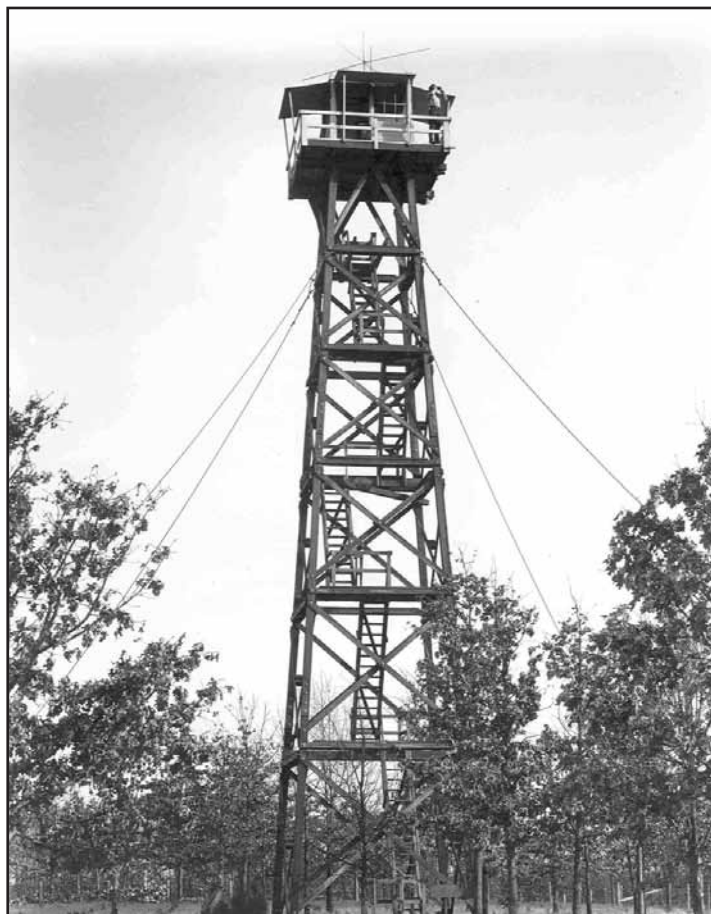
Many of the area's World War Two era fire towers were built of wood due to wartime restrictions on the use of steel. The wooden fire tower at Proctor lasted until replaced by steel in the mid-1970s.
