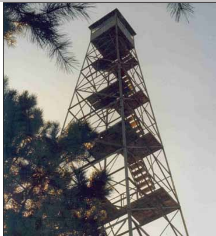
Measuring 80 to 100 feet tall, the galvanized steel towers were fabricated by a windmill manufacturer and assembled on-site, often by MDC crews.
