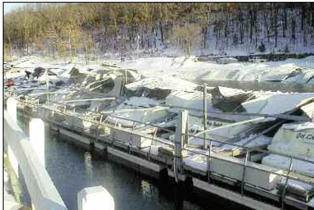
Damage to the docks at Port Arrowhead was extensive under the crushing snow and ice.
