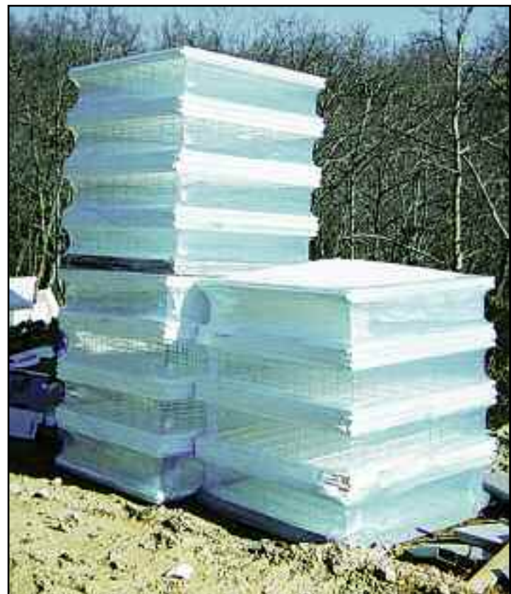
Stacks of ICF panels await placement. ICF panels may someday replace piles of lumber at home construction sites. Gillespie
