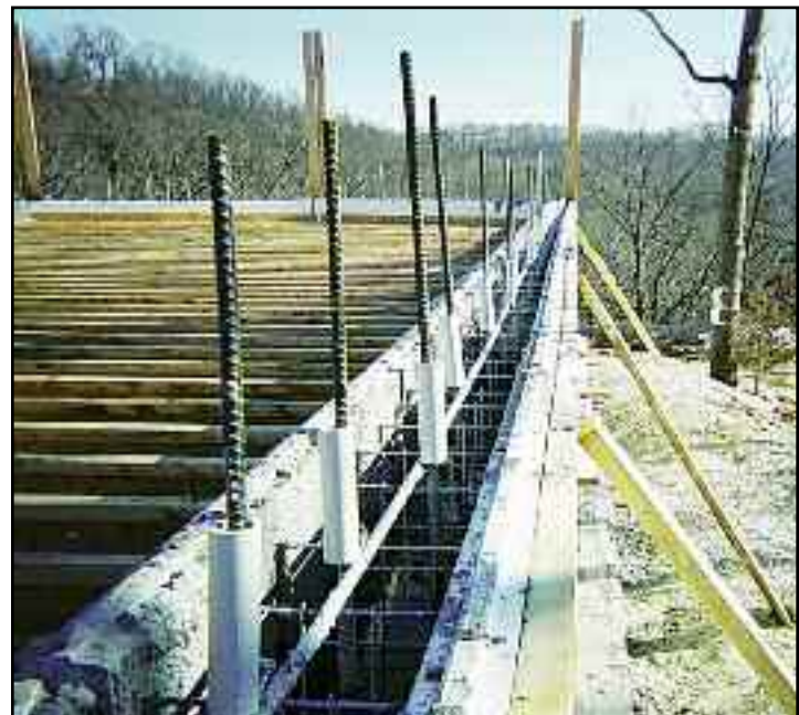
Steel grids and rebar give added strength to the concrete as it dries between the polystyrene forms. Gillespie
