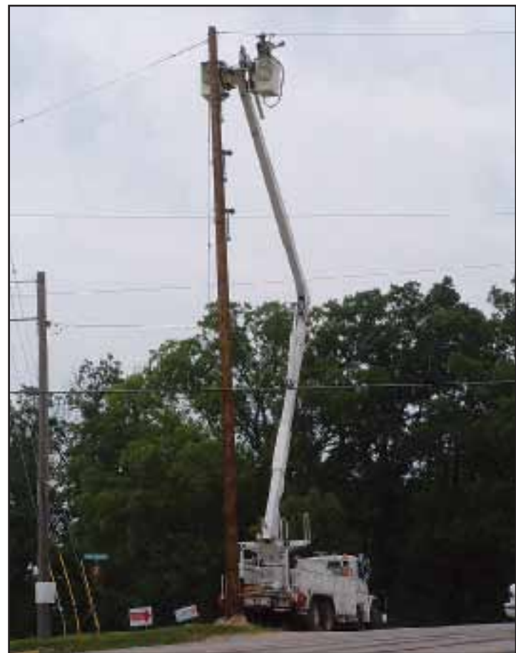
Crews with AmerenUE have been setting poles along Business Route 54. The poles will support new power lines that will be bringing additional electricity to Horseshoe Bend. Nancy Hogland photo.
