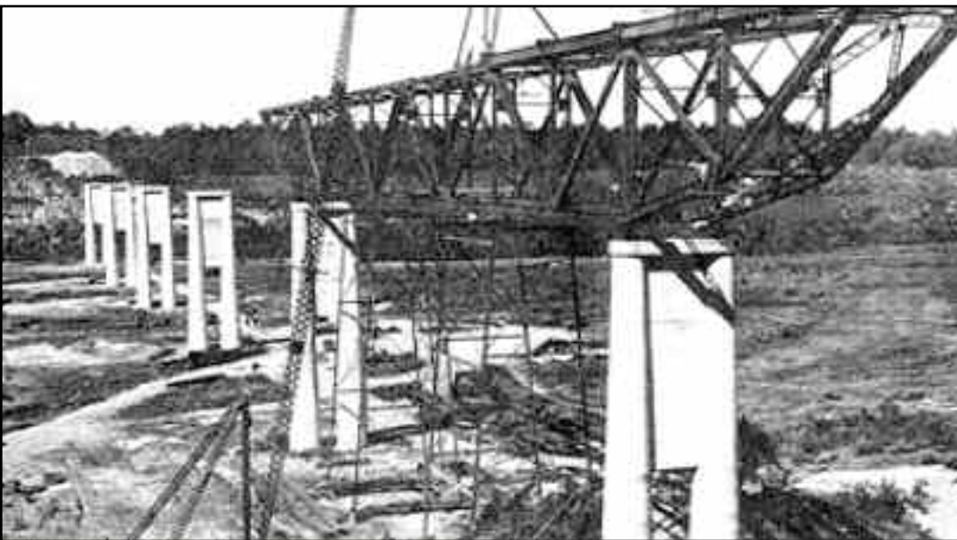
This photo taken in September 1930, looks to the west. The piers were poured during the summer, and now the truss spans are being assembled in place. (Note the temporary support scaffolding under the nearly finished segment.)
