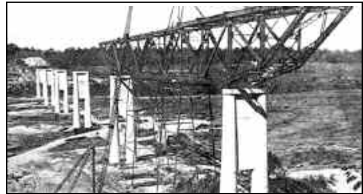
This photo taken in September 1930, looks to the west. The piers were poured during the summer, and now the truss spans are being assembled in place. (Note the temporary support scaffolding under the nearly finished segment.)
