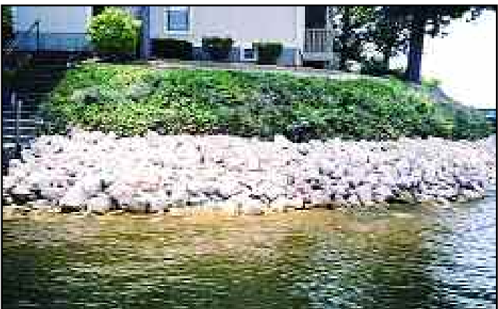
Rip rap protects shores from damaging erosion
