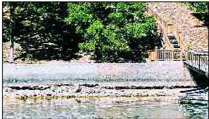
Erosion can eat away at the base of seawalls.
