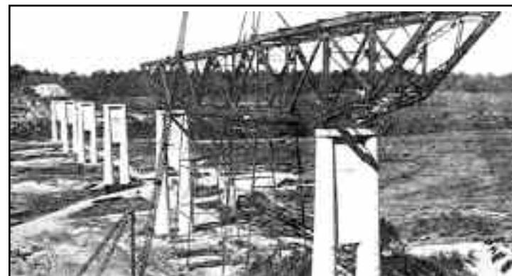
This photo taken in September 1930, looks to the west. The piers were poured during the summer, and now the truss spans are being assembled in place. (Note the temporary support scaffolding under the nearly finished segment.)
